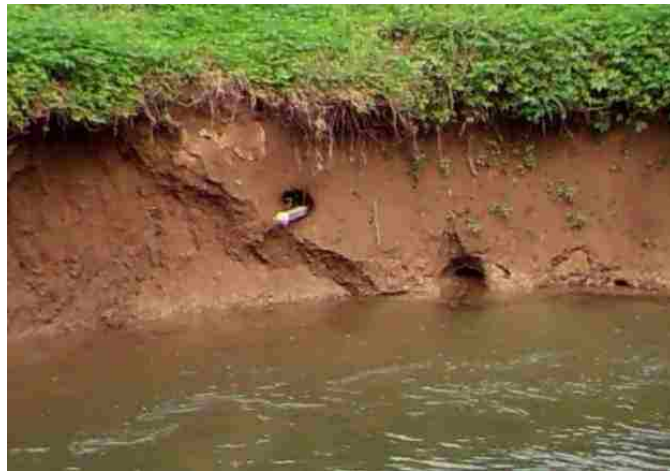
Figure 48. Residual cove formed from drilling
