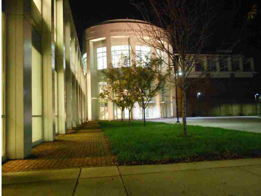
Figure 4.9: Kim Engineering Building, outdoors, front view.
