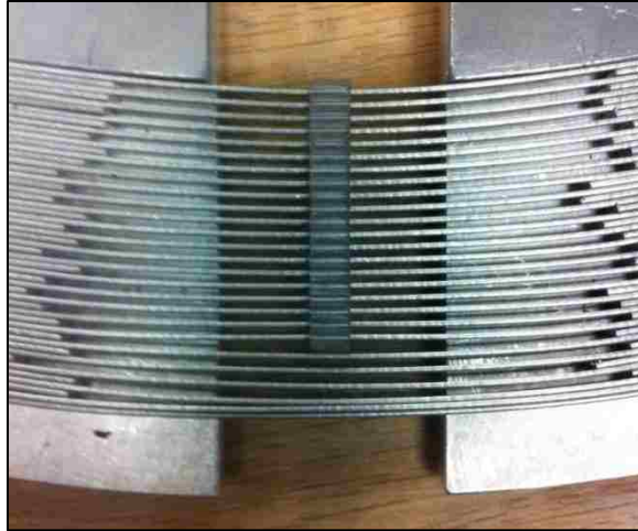
Figure 11 – Short Spacers Removed and Comb Installed into Windings
