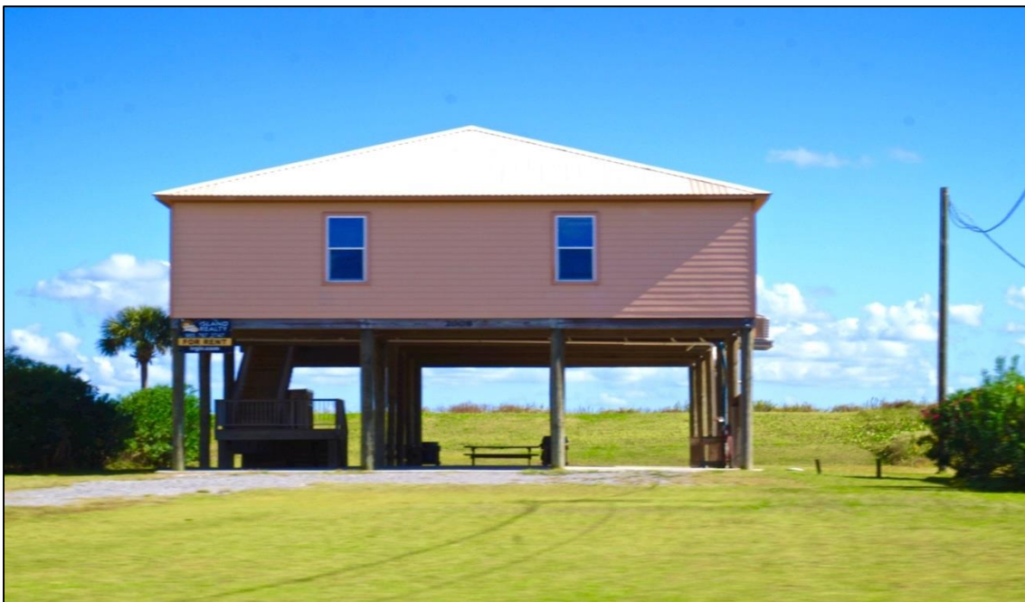
Image 13: Elevated home built behind the hurricane protection dune and overlooking the Gulf of Mexico. Source: Miller, Lauren 2018.
