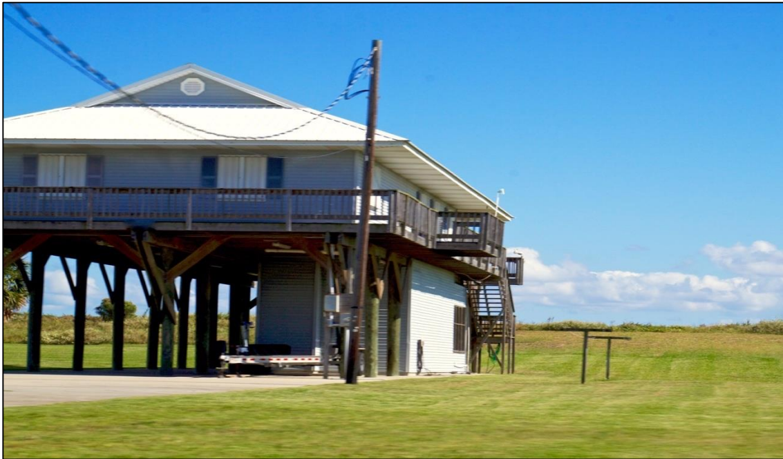
Image 12: Elevated home with storage shed built behind the hurricane protection dune and several pilings supporting the foundation. Source: Miller, Lauren 2018.
