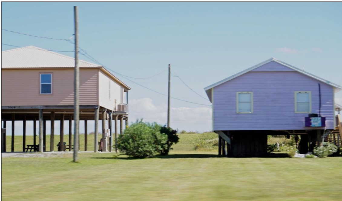
Image 14: House (left) elevated up to code, next door to house elevated according to the older code (right). Both are behind the hurricane protection dune. Source: Miller, Lauren 2018.
