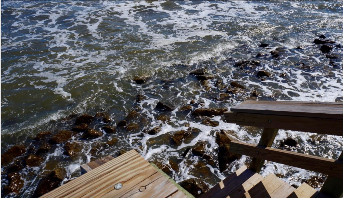
Image 4: HPD and shoreline erosion on the west end of the beach caused waves from the Gulf to come up to this boardwalk. The town placed emergency riprap at this section to halt erosion. Source: Miller, Lauren 2018.
