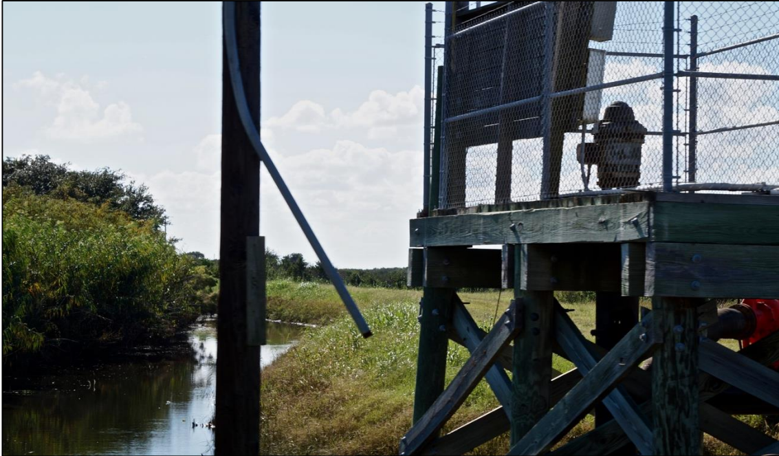
Image 11: Drainage canal (left), tidal surge protection levee (center), and drainage pumps (right). Source: Miller, Lauren 2018.
