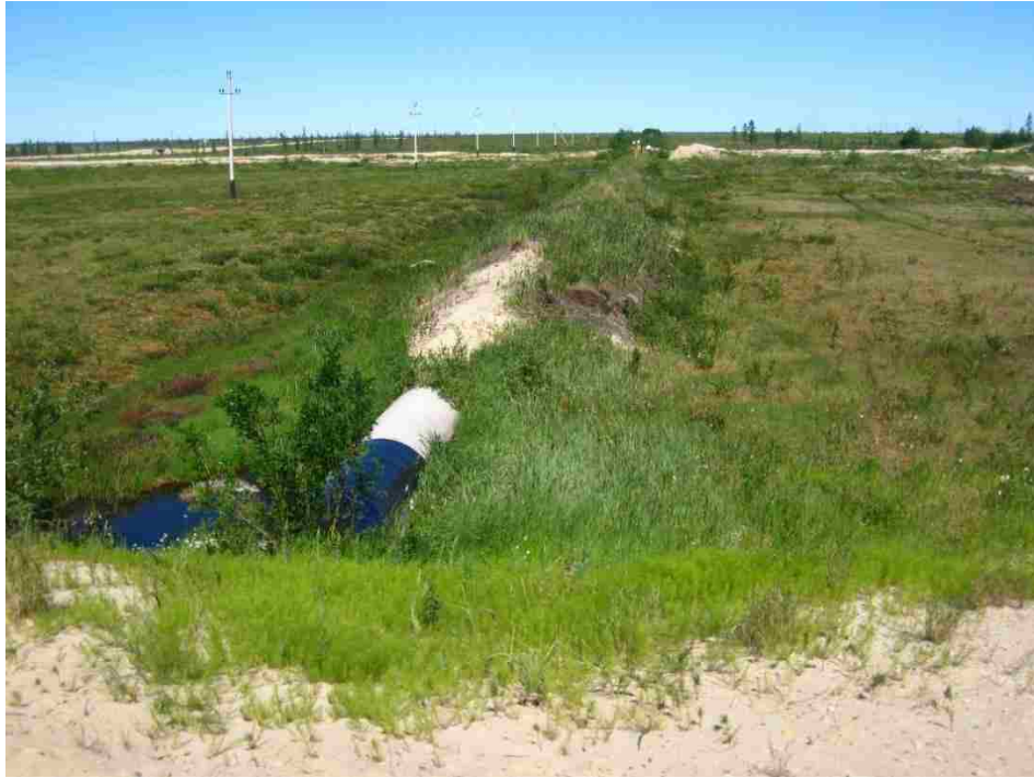
Figure 15. A pipeline buried by locally sourced sand showing revegetation.
