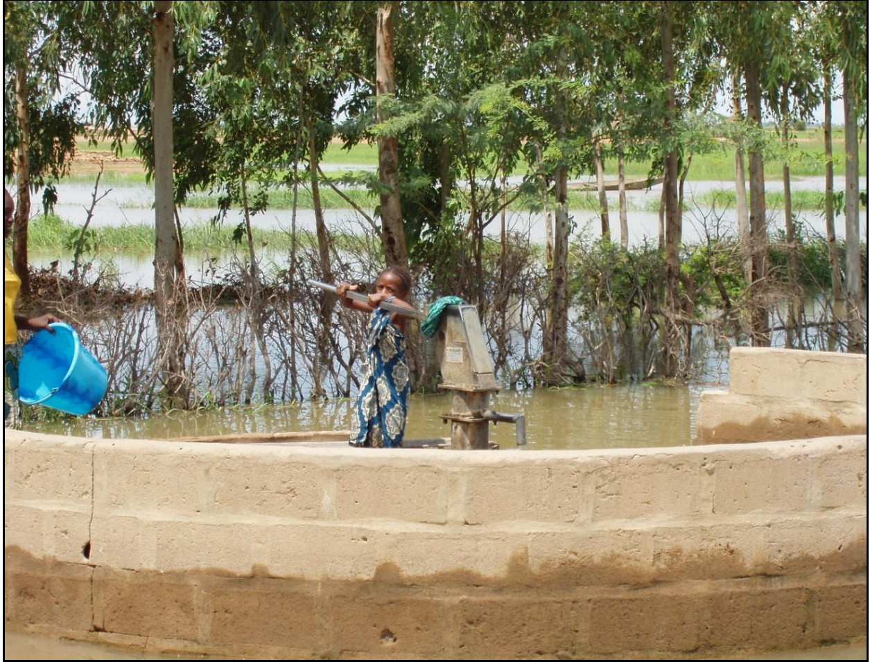
Figure 11. Kobaka was the only village in the study site with a cement encased pump well. This was the only drinking water source that tested negative for E.coli . The well is partially submerged during the Niger River inundation period (Source: Ashley Williams, 2009).
