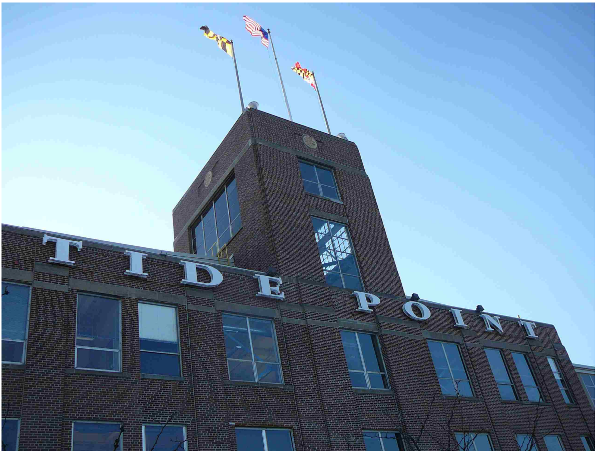
Figure 4. Rejuvenated Tide Point facing Baltimore's Inner Harbor (photo by author)
