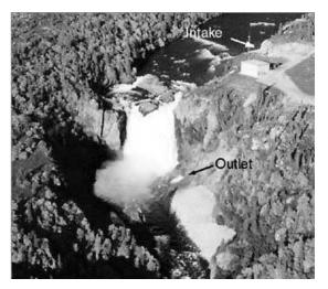
Figure 2. Run of the River Facility (DOE: EERE).
