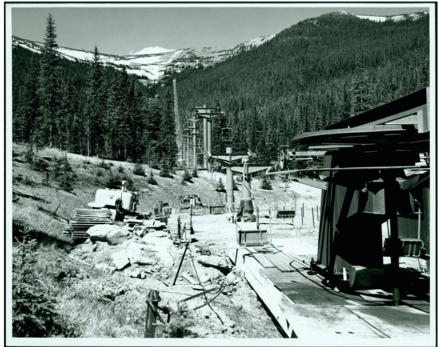
1972. Construction of Hidden Valley chairlift. Photo 2006.013.243, Estes Park Museum.
