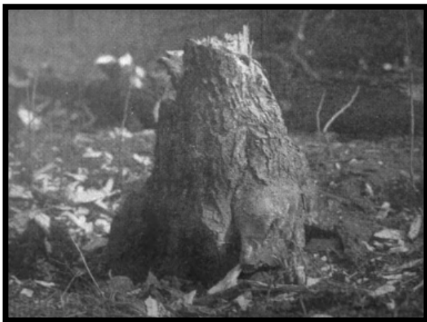
Figure 2: Stump to be blown out with dynamite, circa 1911.
