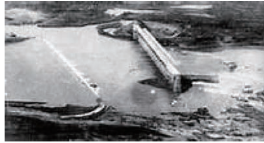
Fig. 1. The Machu Dam failure.
