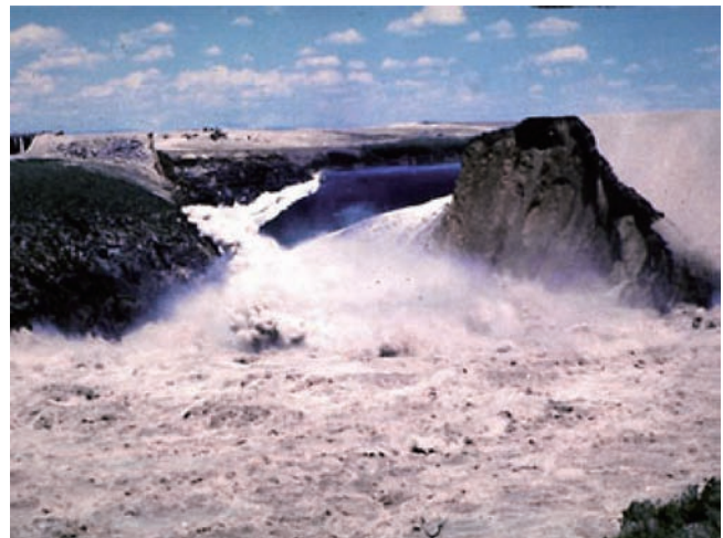
Fig. 9. The Teton Dam failure, 1976 (US).
