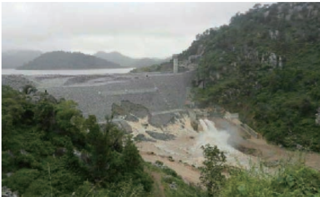
Fig. 8. The failure of the Tokwe Mukosi Dam.
