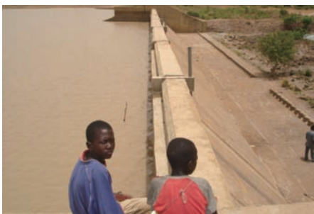
Fig. 5. Concrete fuse plugs for small dams: Wedbila in Burkina Faso.
