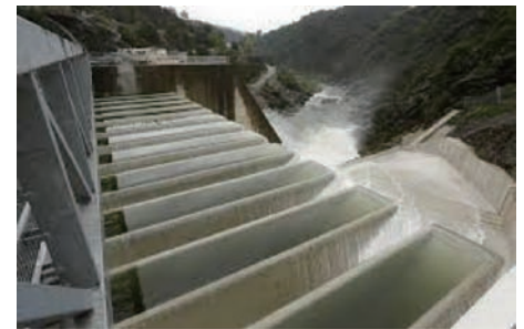
Fig. 4. The Malarce PK Weir in France.
