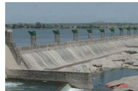
Fig. 6. A flood over the Wanak Bori fuse gates.
