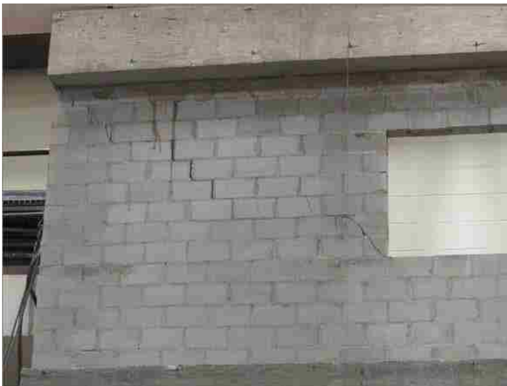
Figure 4-6: Diagonal cracks stepping through mortar joints
