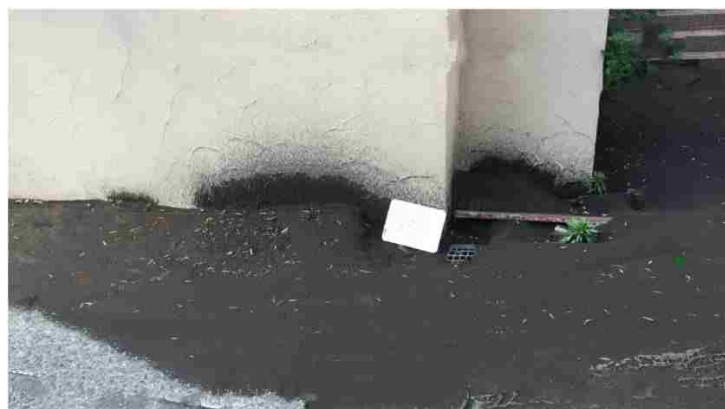
Figure 2-9: Sand boils on side of house in Kumamoto, showing volcanic material that was plastic and pumiceous in origin (Kayen 2017)
