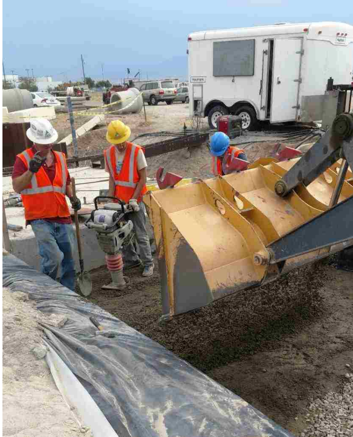
Figure 3-9. Backfill was dumped by backhoe into box, then spread by shovel before compaction.
