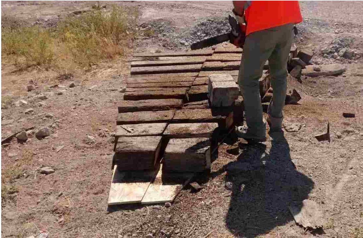
Figure 3-6. Skew wedge base fabrication.
