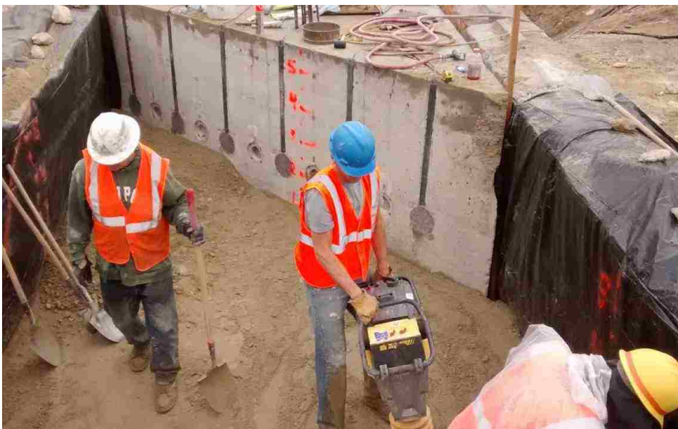
Figure 3-10. Compaction was largely accomplished with use of jumping jack compactors.
