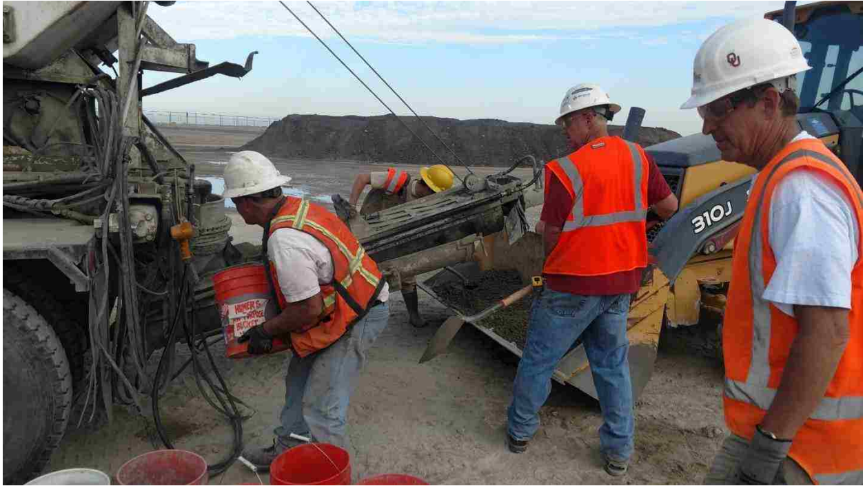
Figure 3-8. For 0° test, extra aggregate was added to each batch in order to meet cement content requirement.
