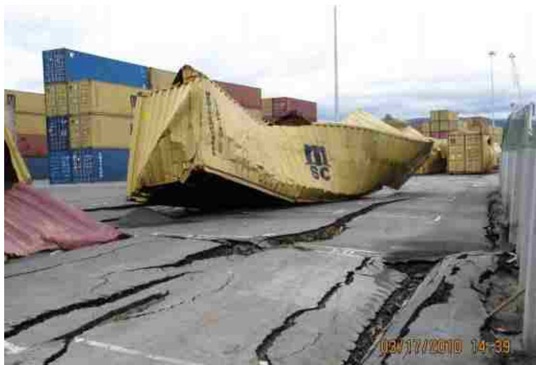
Figure 6-6: Toppled Containers at the Port of Coronel (GEER 2010)
