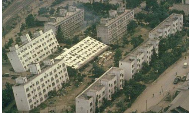
Figure 2-11: Example of Bearing Capacity Failure During the 1964 Niigata, Japan Earthquake (Photo from quakeinfo.ucsd.edu/ )
