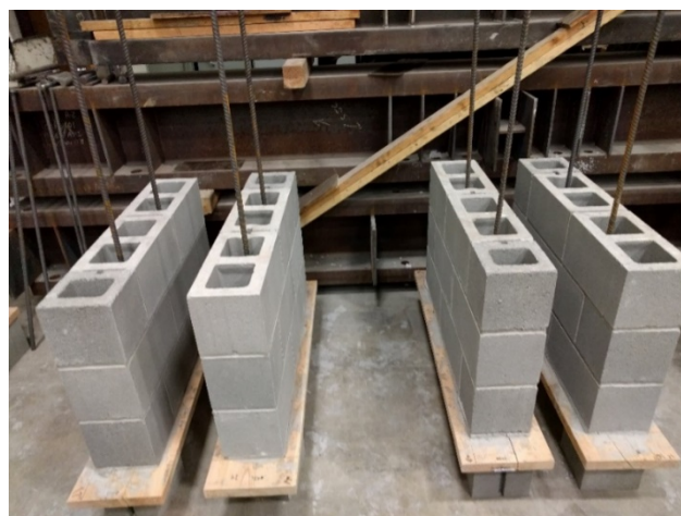
Figure 3-5: Panels Before Grouting
