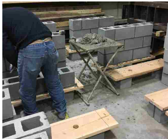
Figure 3-4: Masonry Panel Construction
