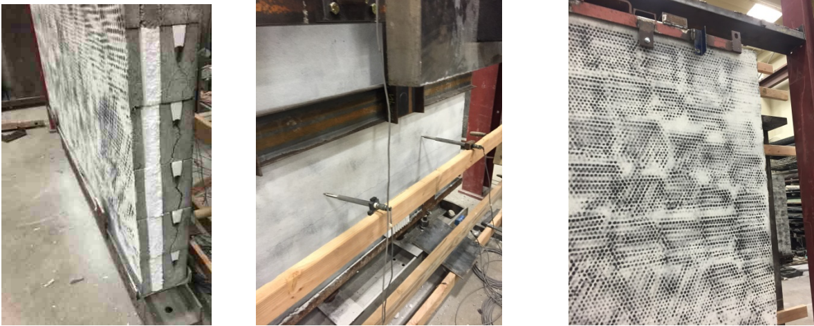
(a) Cracking in webs. (b) Cracking at bottom of wall. (c) No visible cracks in top of wall.
