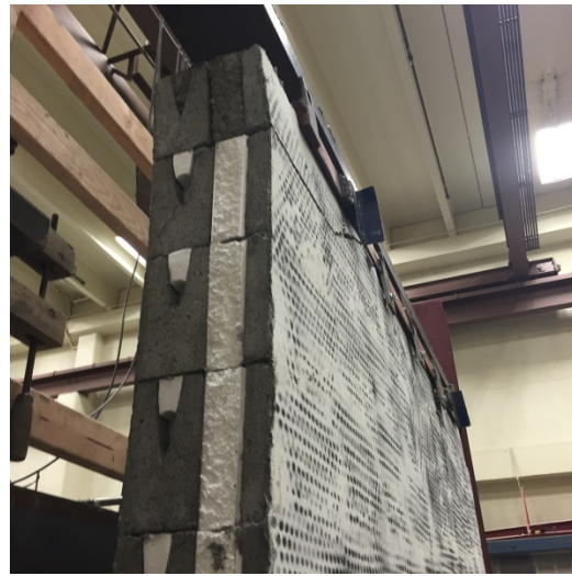
(b) Crack through top course.
