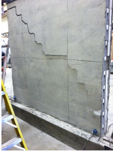
(b) Diagonal crack.
