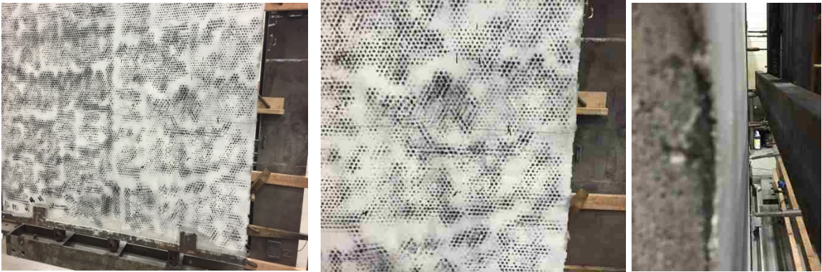
(a) Overall view.
