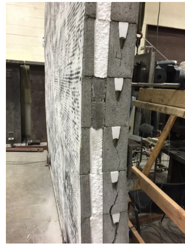
(c) Cracking through webs.
