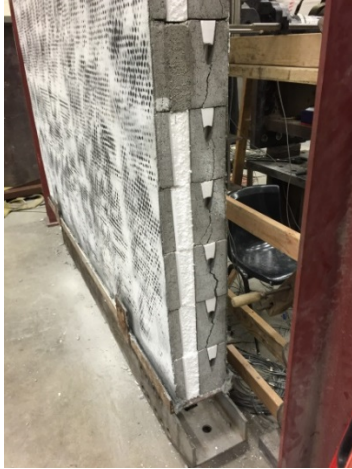
(a) Cracks in webs.
