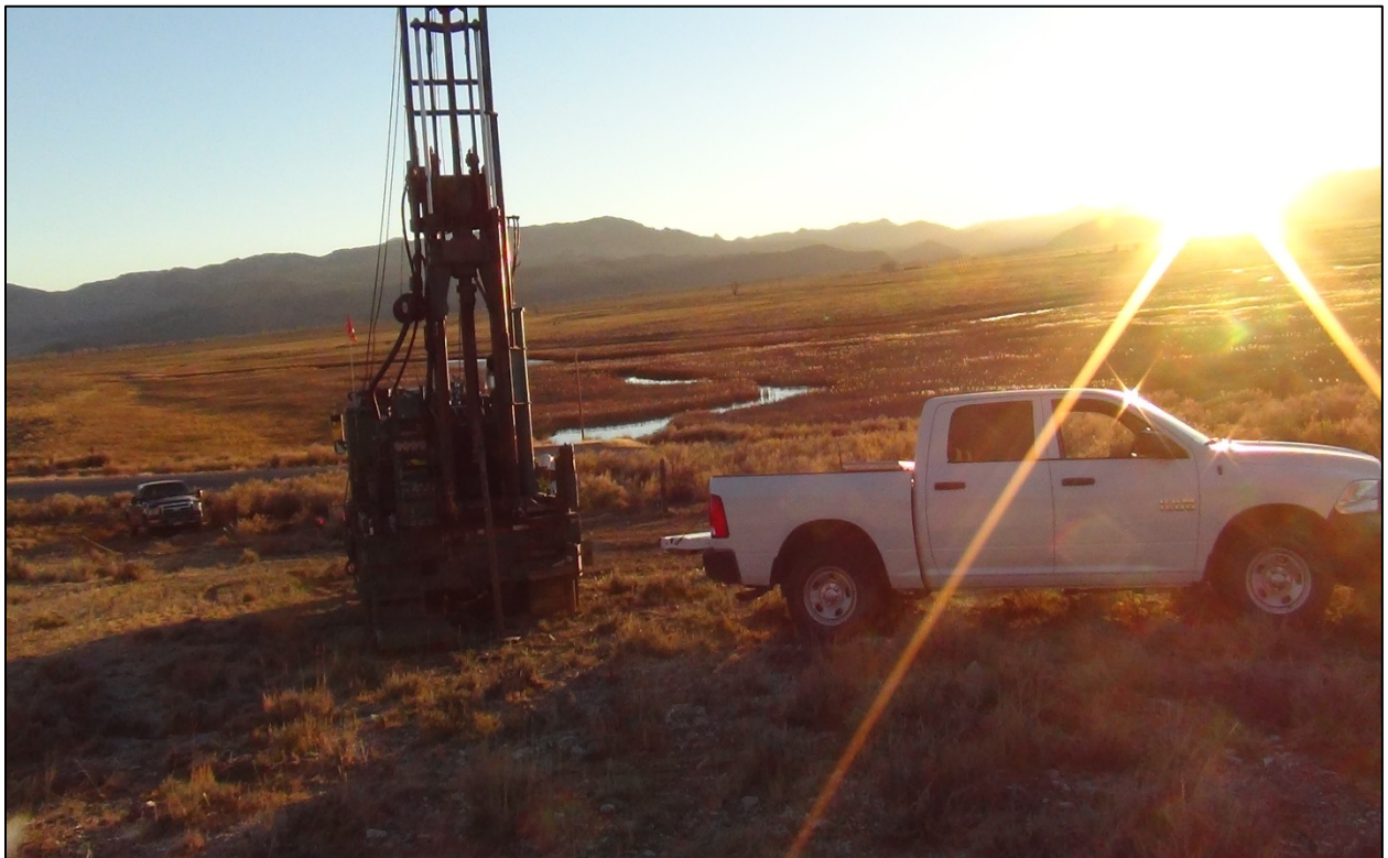
Figure 6-7. Photograph showing site conditions at Whiskey Springs in 2015 near BC3, looking southwest. Highway 93 can be seen in the background.
