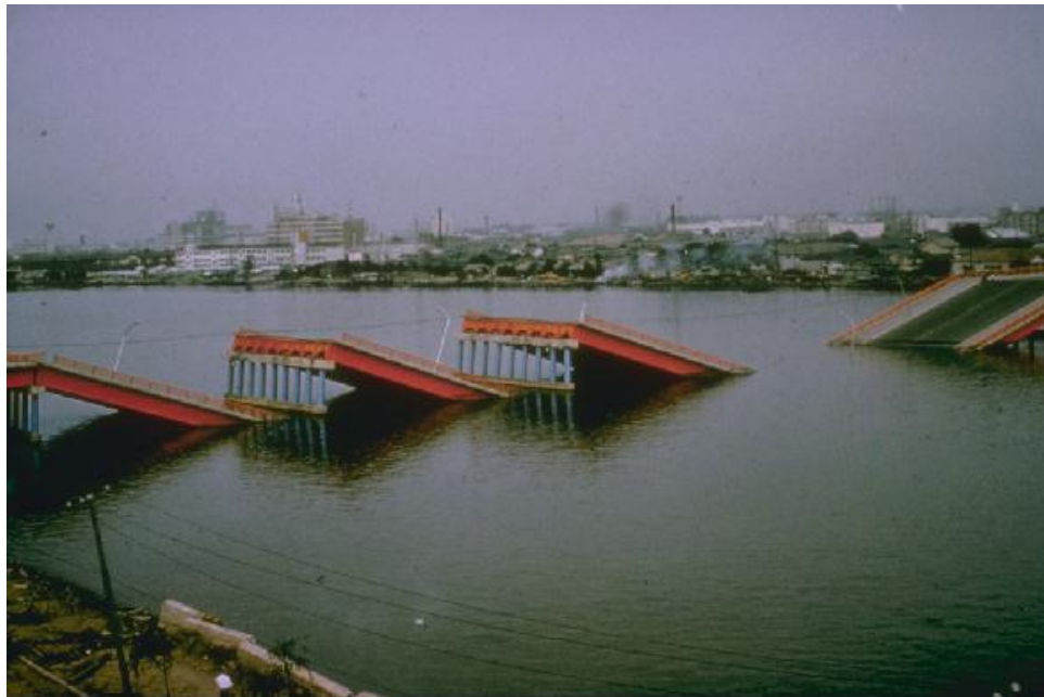
Figure 1-1 Lateral Spread Collapsed the Showa Bridge, Niigata, Japan. The City Suffered Slight Damage from Shaking, But Heavy Damage from Liquefaction (NRC, 1985).
