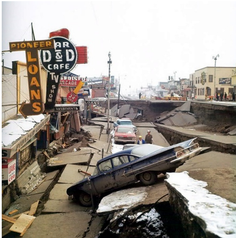
Figure 1-2 Downtown Anchorage, AK Experienced Flow Deformation and Lateral Spreading Which Caused Downhill Slumping Towards the Harbor as a Result of Liquefaction Caused by M_w 9.2 Earthquake of 1964.
