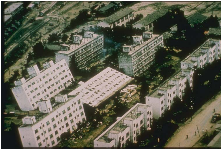
Figure 3-14: Bearing capacity failure of structures from soil liquefaction in Niigata, Japan (1964) (after NOAA/NGDC - NOAA National Geophysical Data Center).
