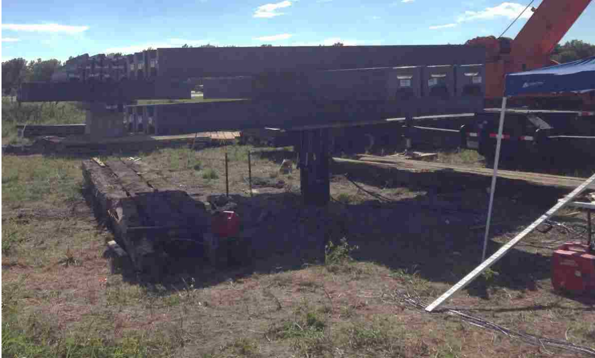
Figure 4.4-8 Photo of the loading configuration completed.
