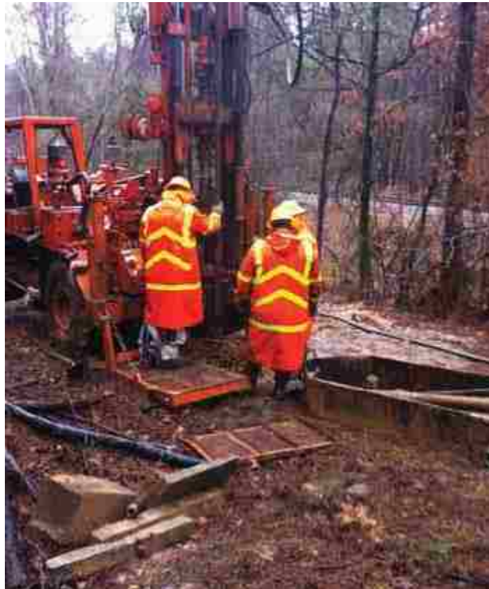
Figure 3.1-3 Photo of the drill rig for the standard penetration test (SPT) (Bey 2014).
