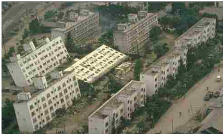
Figure 3-21: Apartment buildings after the 1964 Niigata, Japan earthquake.
