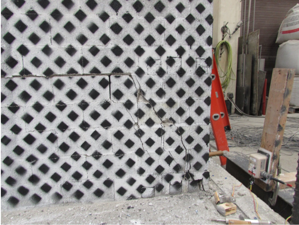
Figure 3-18: Cracking Through the Grouted Cells
