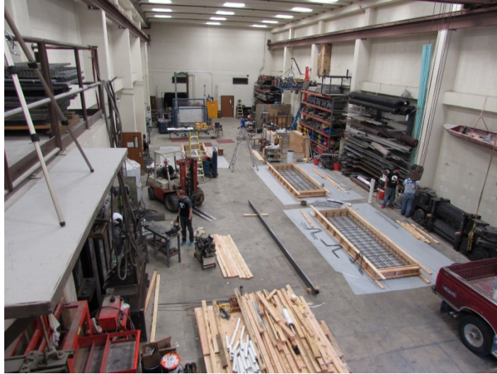
Figure 3-4: Footing Reinforcement Cages and Forms
