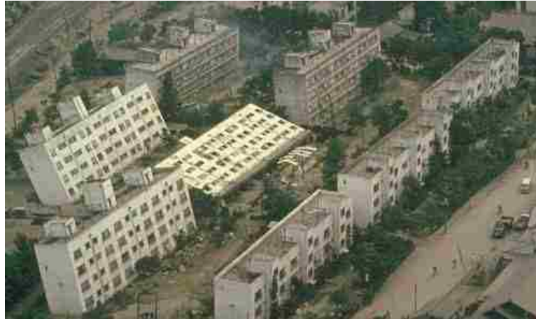
Figure 3-21: Example of a loss of bearing capacity failure causing apartment buildings to collapse in Niigata, Japan, after the 1964 earthquake (after Kramer (1996)).
