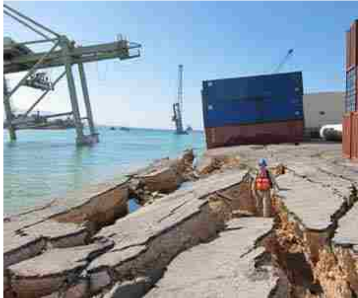
Figure 4-2: Example of lateral spread displacements causing fissures along a port in Haiti after the 2010 earthquake (after Eberhard et al. (2013)).
