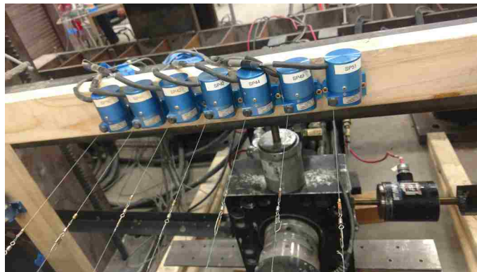
Figure 3-8 : String potentiometers mounted on independent wooden reference frame to monitor longitudinal deflection of the LCC backfill surface.
