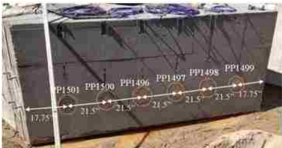
Figure 3-11: Photograph of embedded pressure plates showing horizontal spacing dimensions
