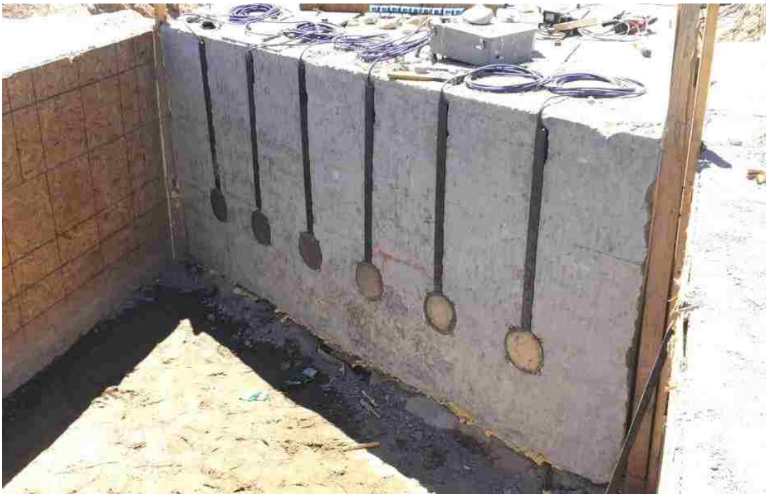
Figure 3-12: Photograph of pressure plates and steel channels on skew wedge
