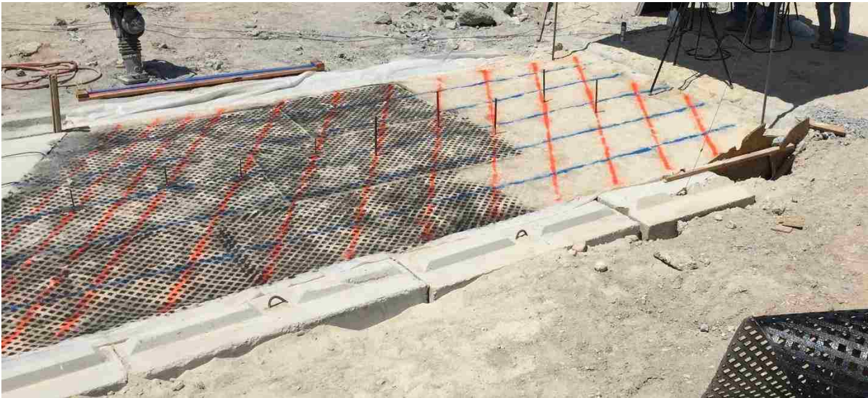
Figure 4-5: Photo of the grid line layout for the 30° skew test
