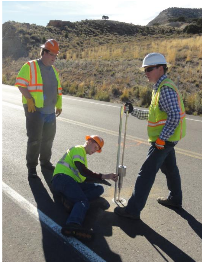
Figure 3-3: DCP testing of pavement structure.
