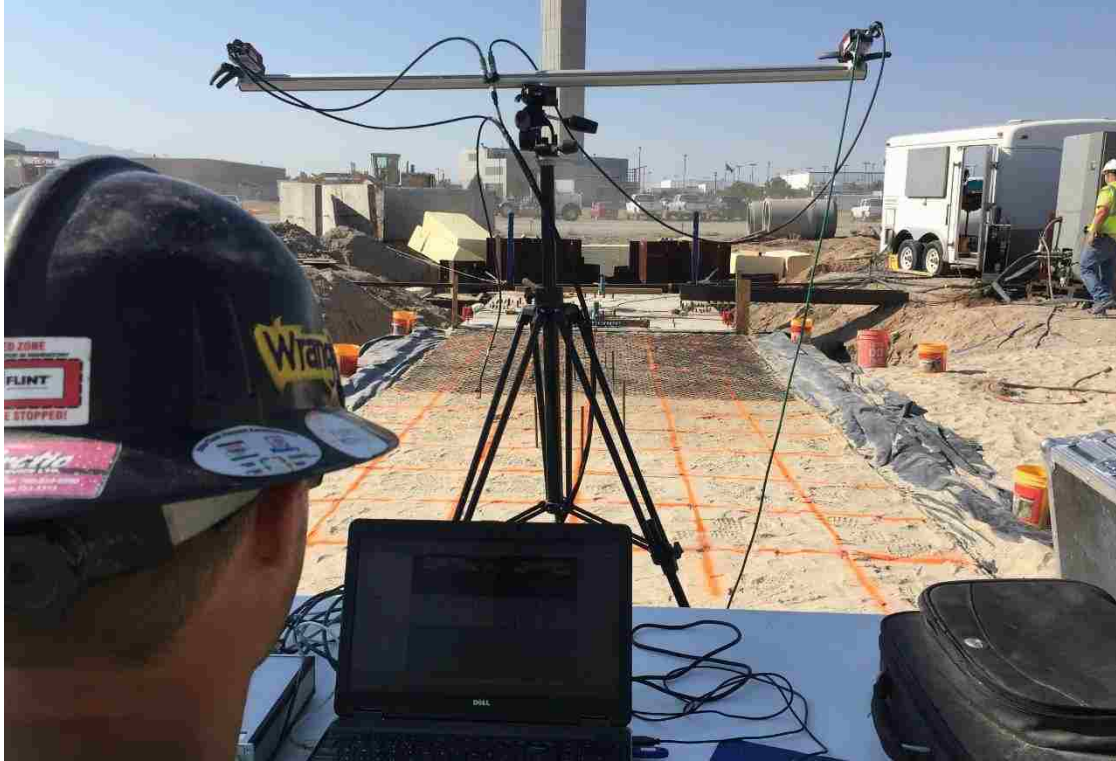
Figure 3-9: DIC cameras on tripod just past the north edge of the backfill
