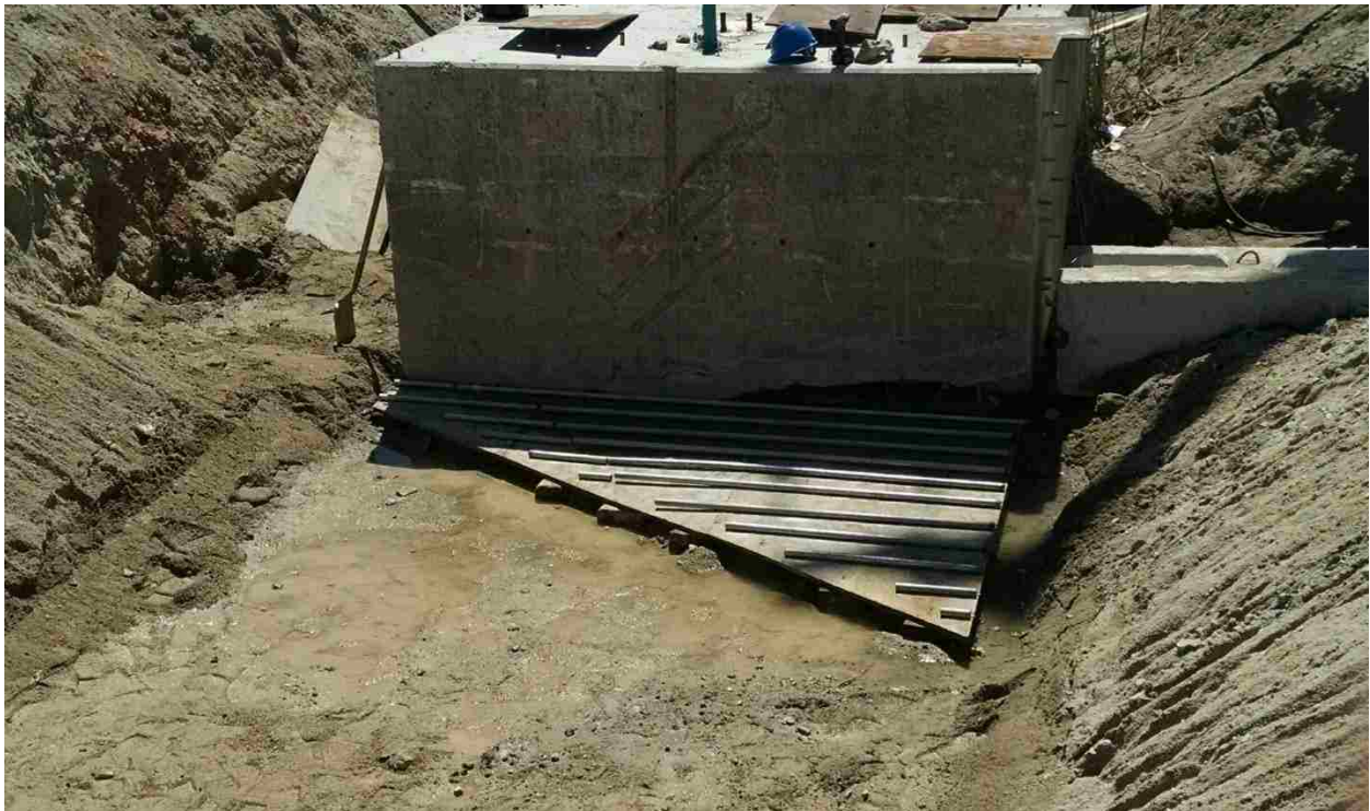
Figure 3-5: Skew wedge base composed of railroad ties, 0.75-inch plywood, and rollers
