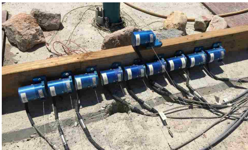
Figure 3-7: String potentiometers mounted on the pile cap
