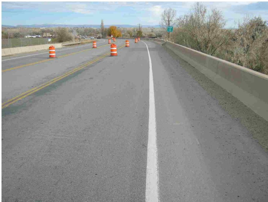
Figure 2-6: Deck with asphalt overlay.
