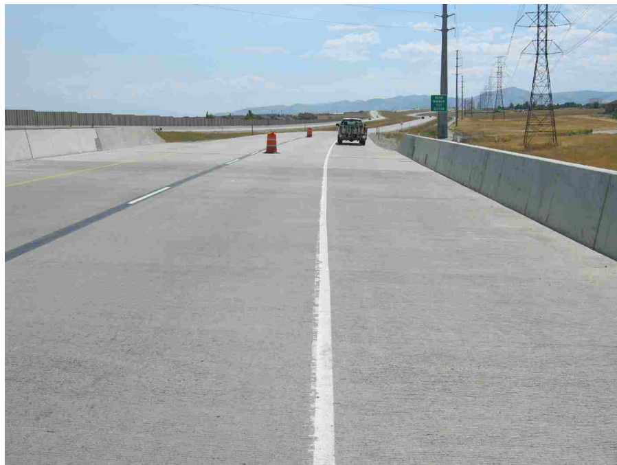
Figure 1-1: Bare concrete bridge deck.
