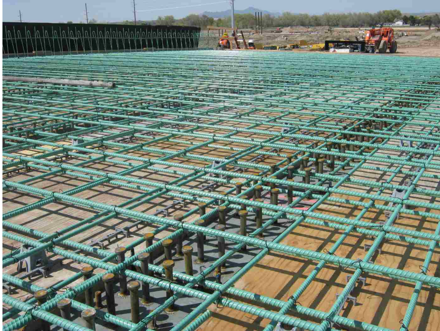
Figure 2-5: Epoxy-coated reinforcement.
