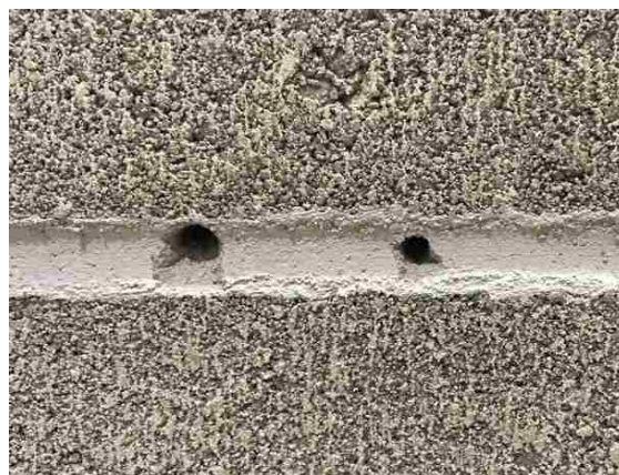
Figure 3-9: Original Helix Hole and Secondary Pilot Hole
