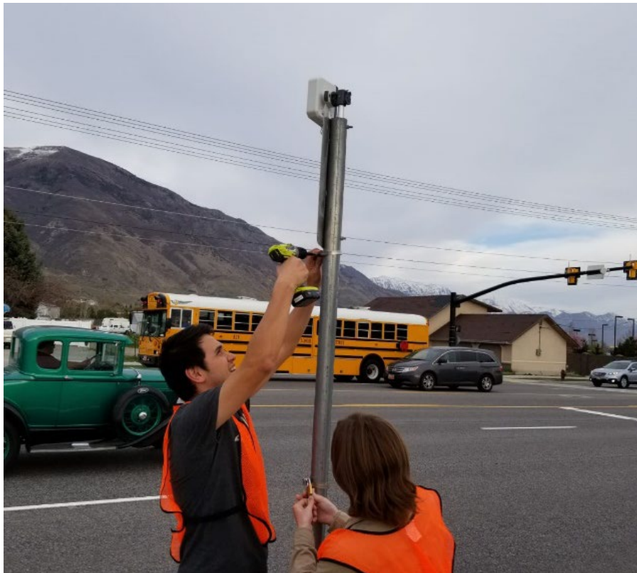
Figure 3-2: Research Assistants Mounting a COUNTCam2 Camera
