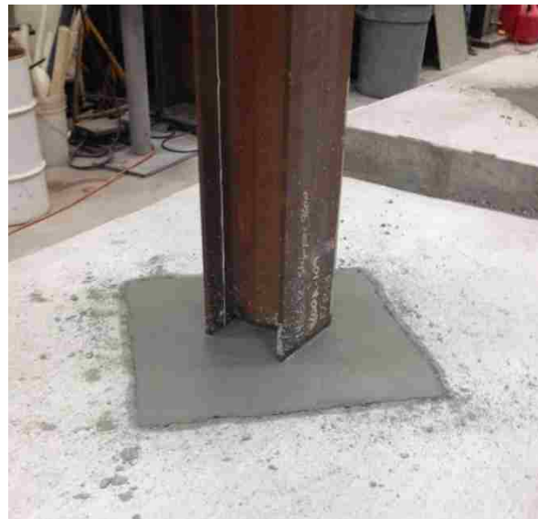
Figure 2.13: Shallow Embedded Column Specimen After Block-Out Pour (Barnwell)
