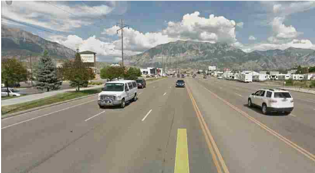
Figure 5-20:View of 800 North at 480 West, Orem (Google Earth, 2015).
