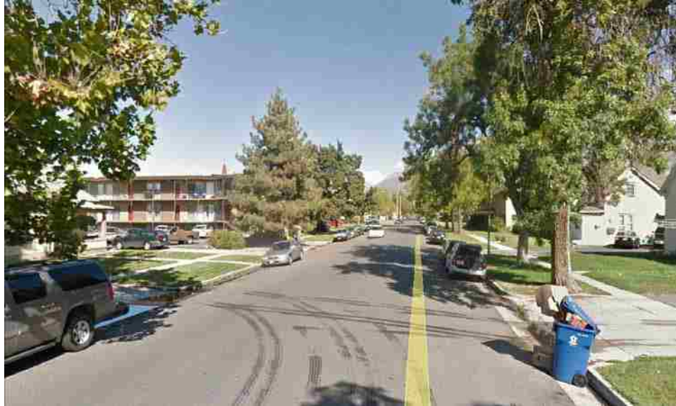
Figure 5-43: View of 100 East at 450 North, Provo (Google Earth, 2015).
