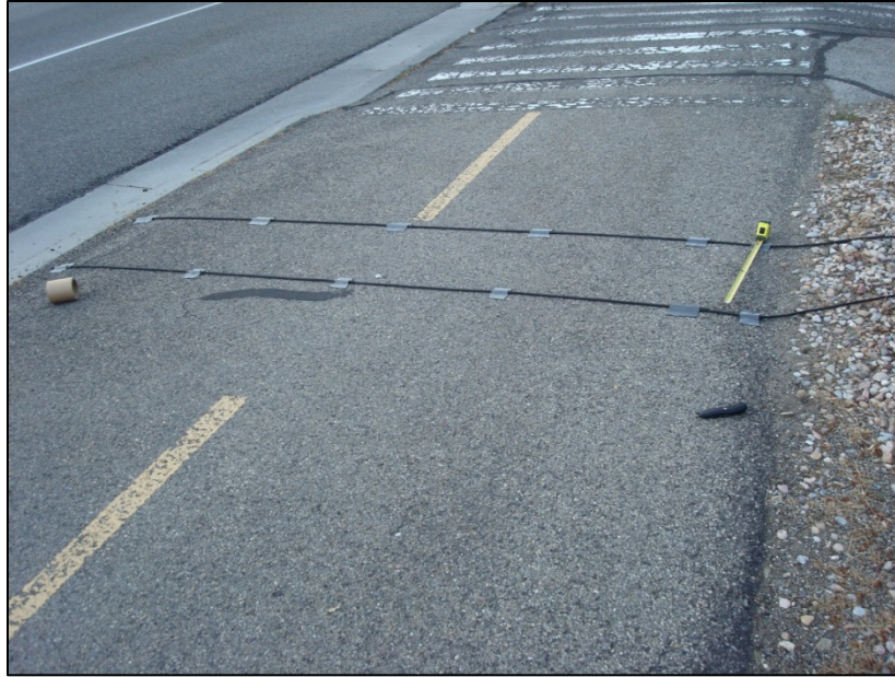
Figure 4-7: Placement of mini tubes (photo taken by Chris Haskell, 2015).
