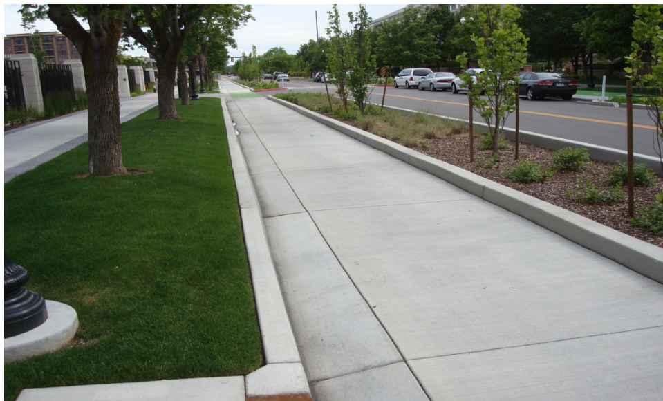
Figure 5-53: View of Grant Ave at 2125 South, Ogden (photo taken by Chris Haskell, 2015).
