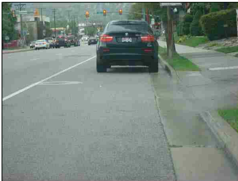
Figure 5-12: Southbound view of the paved shoulder at 700 East at 550 South, Salt Lake City (photo taken by Chris Haskell, 2015).
