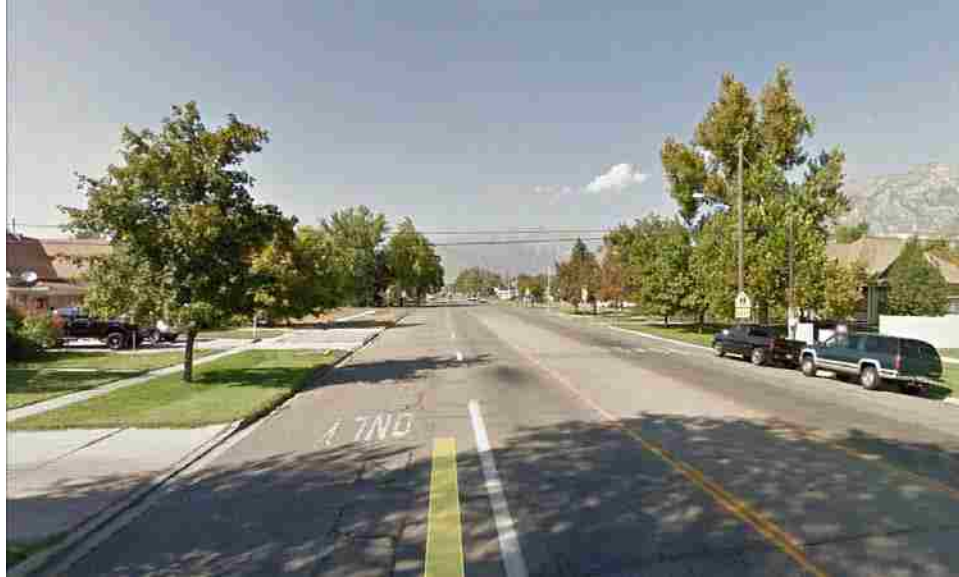
Figure 5-39: View of 500 West at 450 South, Provo (Google Earth, 2015).
