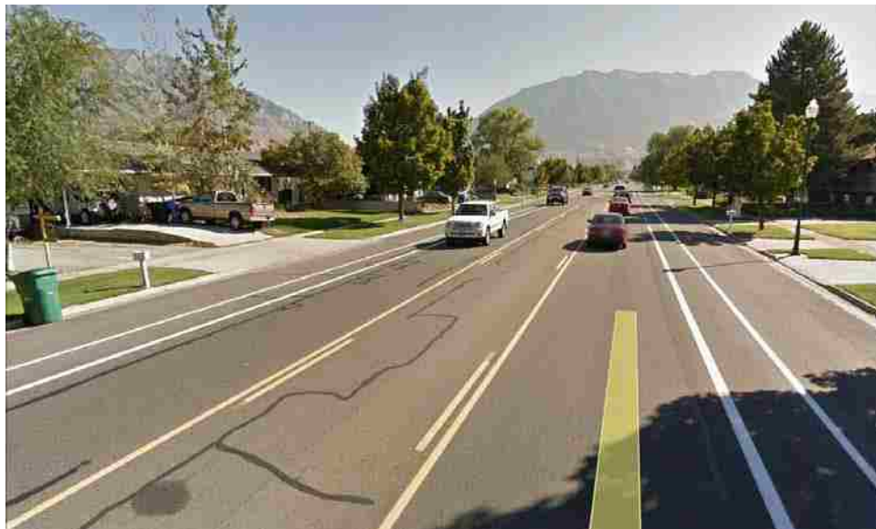
Figure 5-22: View of 400 North at 350 West, Orem (Google Earth, 2015).
