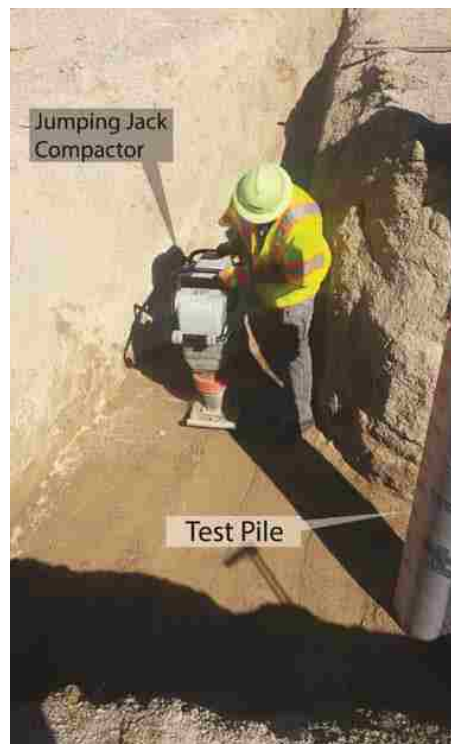
Figure 3-8: Jumping Jack Compactor in Phase 3 of Compaction.
