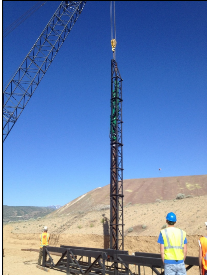
Figure 3-3: Installation of piles using a diesel hammer.
