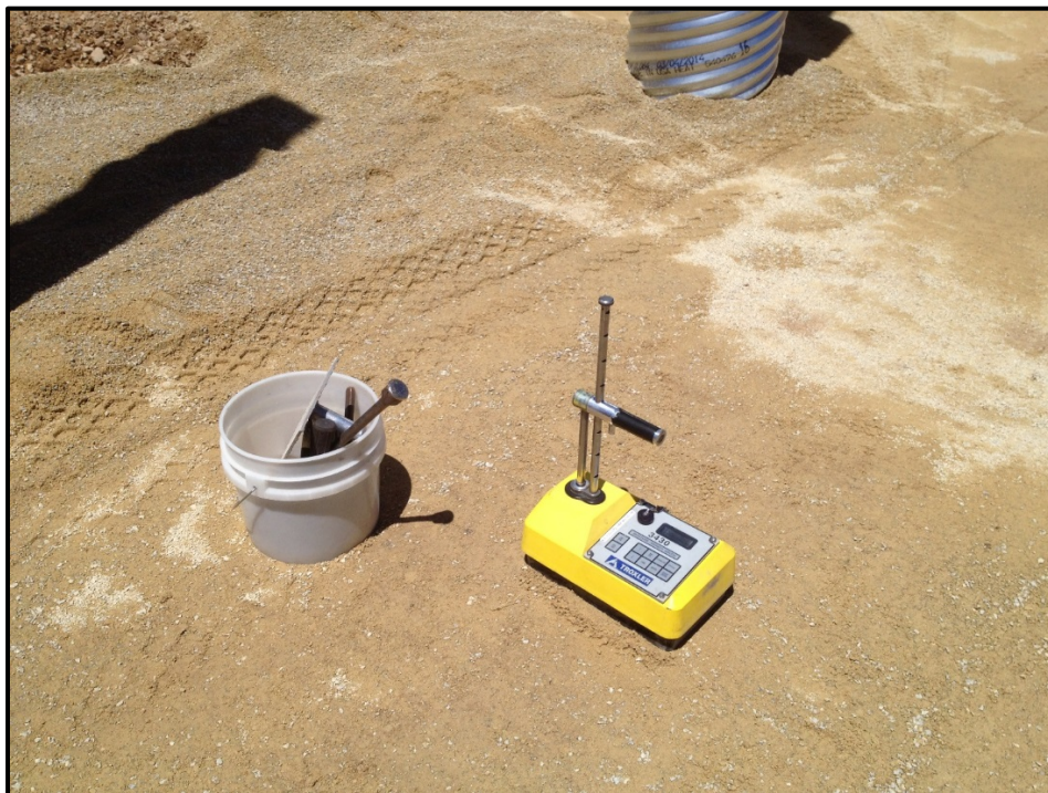
Figure 3-14: Density and moisture testing of backfill using a nuclear density gauge.
