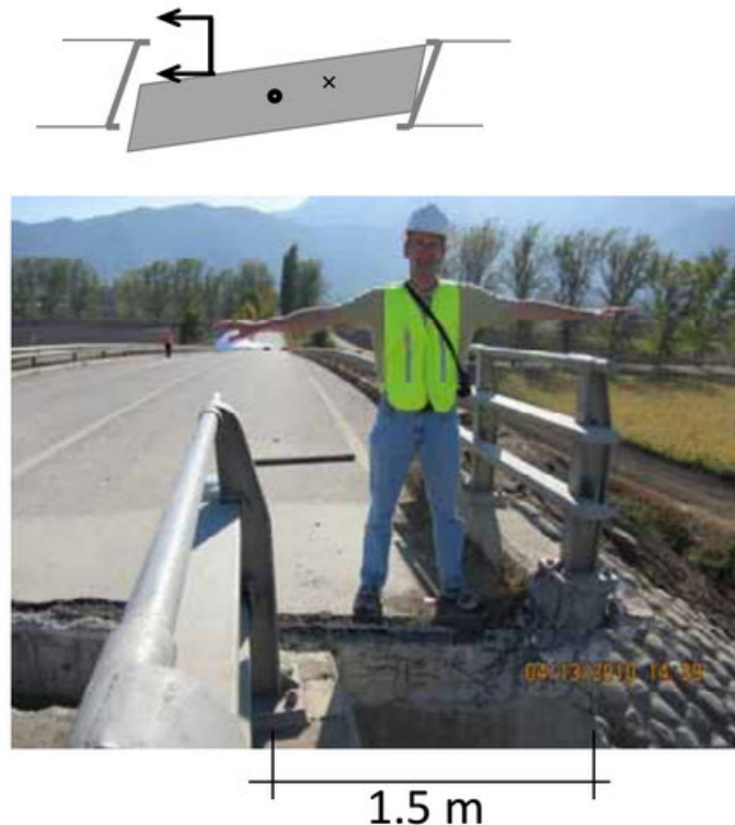
Figure 2-19. Bridge superstructure translation (Elnashi et al. 2010).
