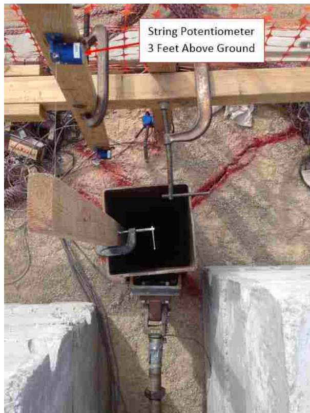
Figure 4-2. String potentiometer attached three feet above the pile.
