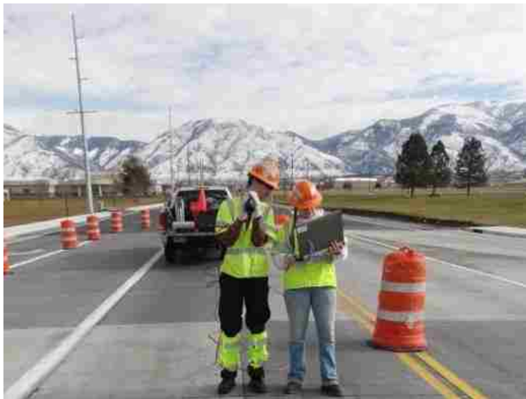
Figure 3-10: Measurement of surface temperatures using infrared thermography.
