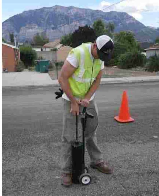
Figure 3-17: CIST testing of base layer.
