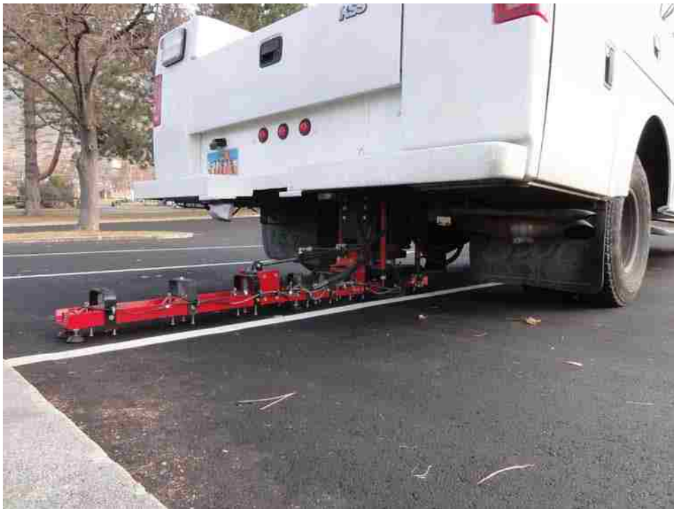
Figure 3-20: FWD testing of pavement.
