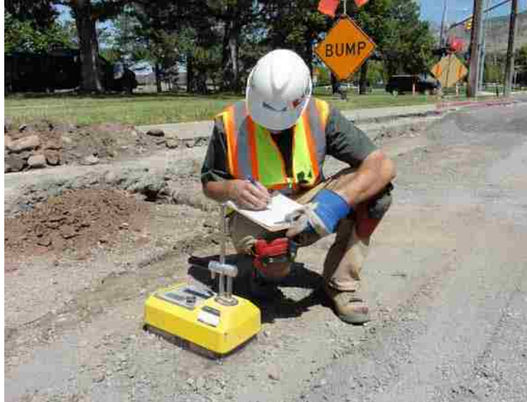
Figure 3-14: NDG testing of subgrade.
