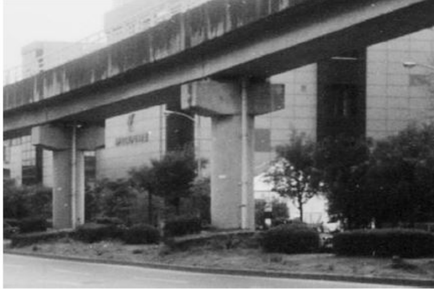
Figure 5-2: Example of ground elevation change from settlement (after Tsukamoto and Ishihara 2010)
