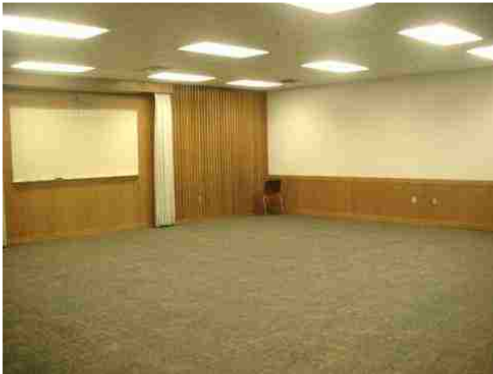
Figure 3.5 A conference room with dimensions 9.3 x 9.2 x 2.7 and volume 231 m 3 . The floor is carpeted cement, the walls are made of wood paneling and drywall, and the ceiling is composed of suspended acoustic tiling.
