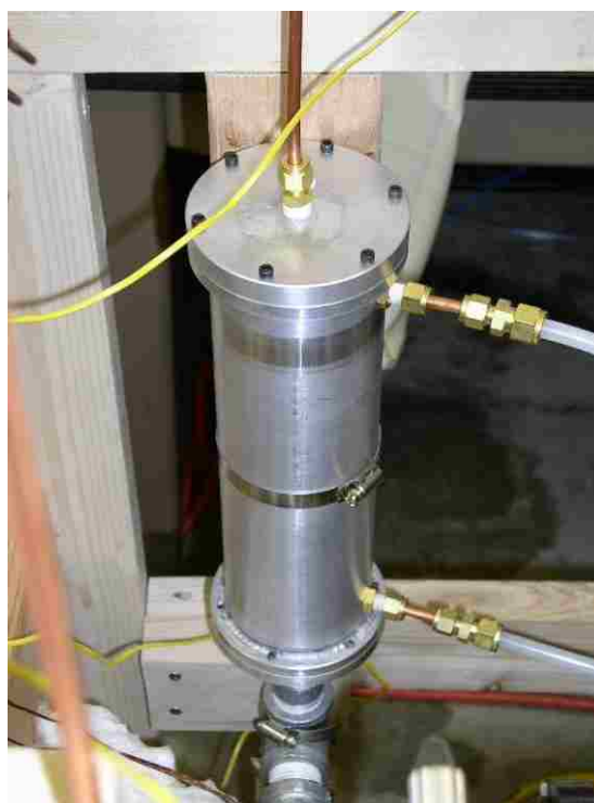
Figure 12. Heat exchanger (E-103) used to cool CO gas and condense water vapor.
