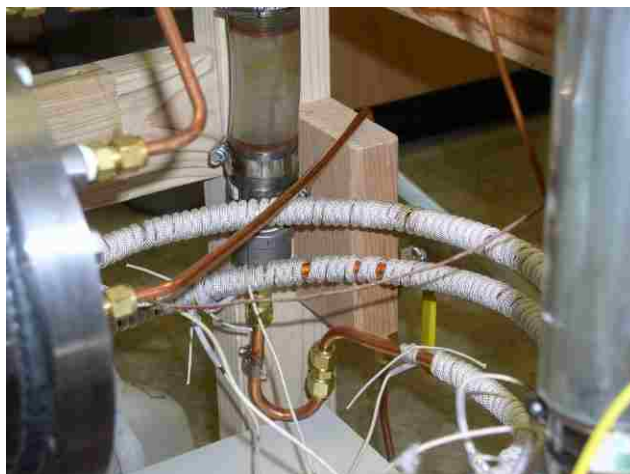
Figure 26. Sight tube at the bottom of the column, above “p trap”
