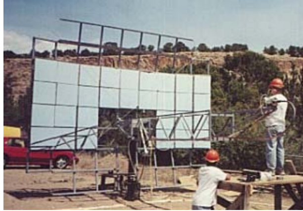
Figure 2-2. Photo of the solar collector and CO 2 converter device.
