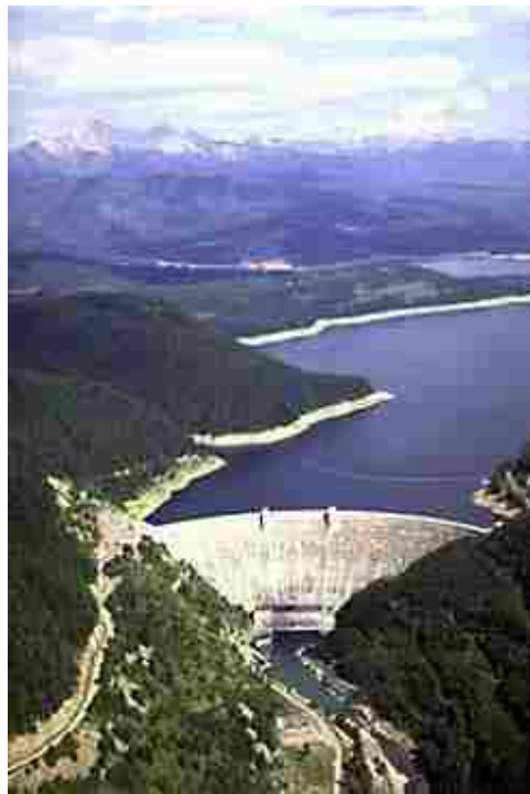
Figure 1-2 Hungry Horse Dam built with fly ash concrete in Montana, USA ( http://www.usbr.gov/dataweb/dams/mt00565.htm )
