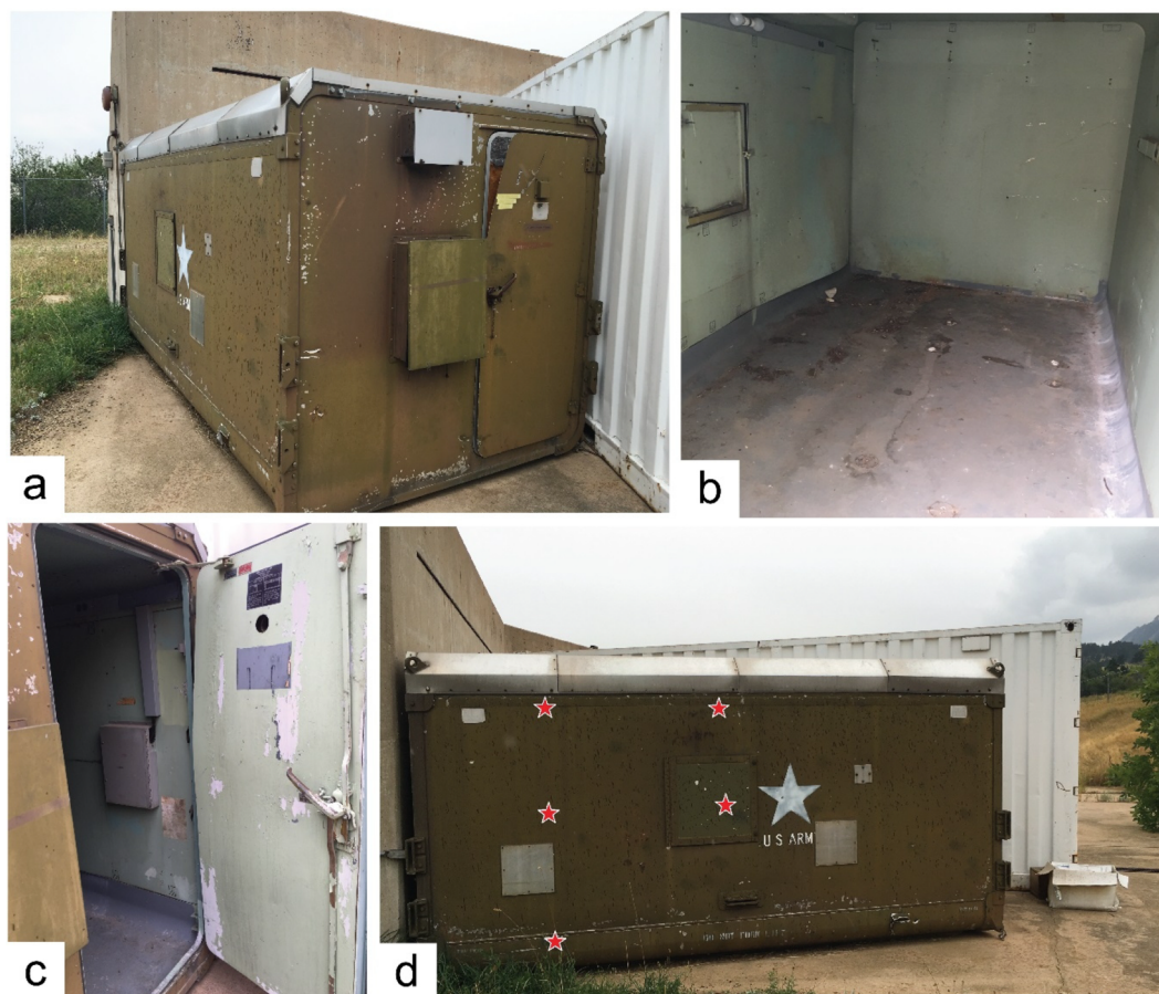
Fig. 1. Photographs of the bunker are presented. (a) Exterior front and side of the bunker. (b) Bunker interior. (c) Open hatch on the front wall. (d) Side view of the bunker; one of the walls into which sampling ports were drilled. Port locations are indicated with ★.
