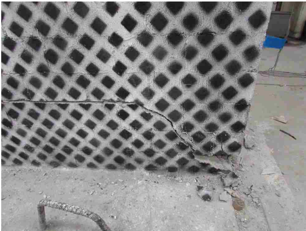
Figure 4-14: Toe crushing of experimental masonry wall
