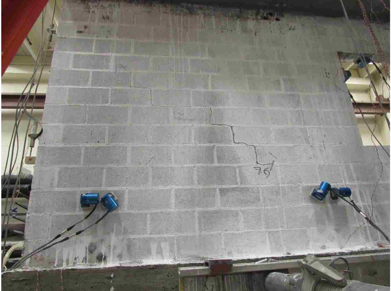
Figure C-3: Enlarged view of 2 nd story cracks in push regime
