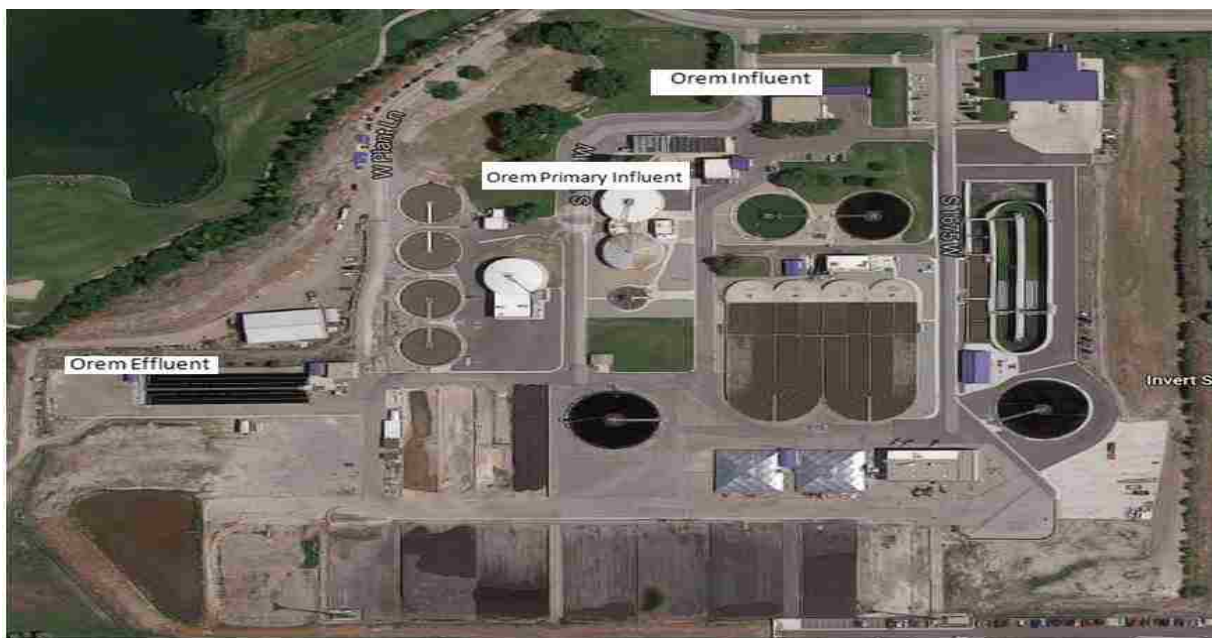
Figure 3-3 Aerial View of the Orem Waste water Treatment Plant
