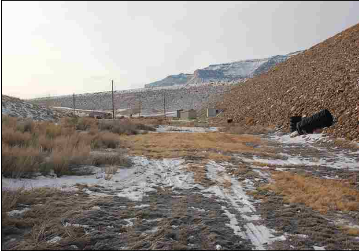
Figure 8-4. View of conditions and topography at Millsite Dam, looking south along the downstream toe of the dam, January 2015.
