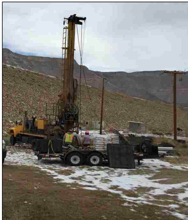
Figure 8-3. View of drill rig used at Millsite Dam looking north along the downstream toe of the dam, January 2015.
