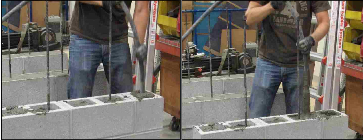
Figure 19. Consolidation of Grout using Vibratory Stinger
