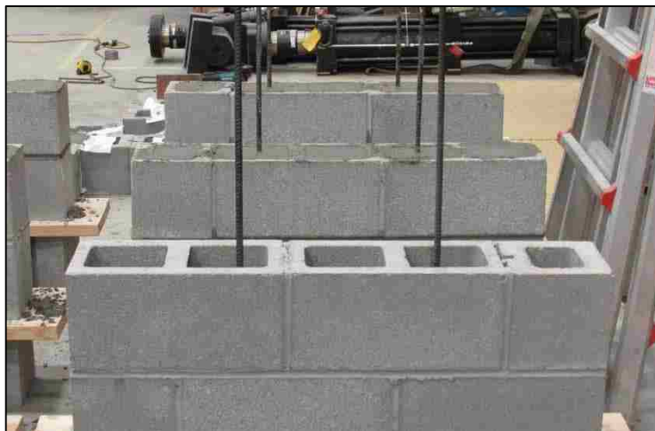
Figure 16. Placement of Reinforcement Prior to Grouting
