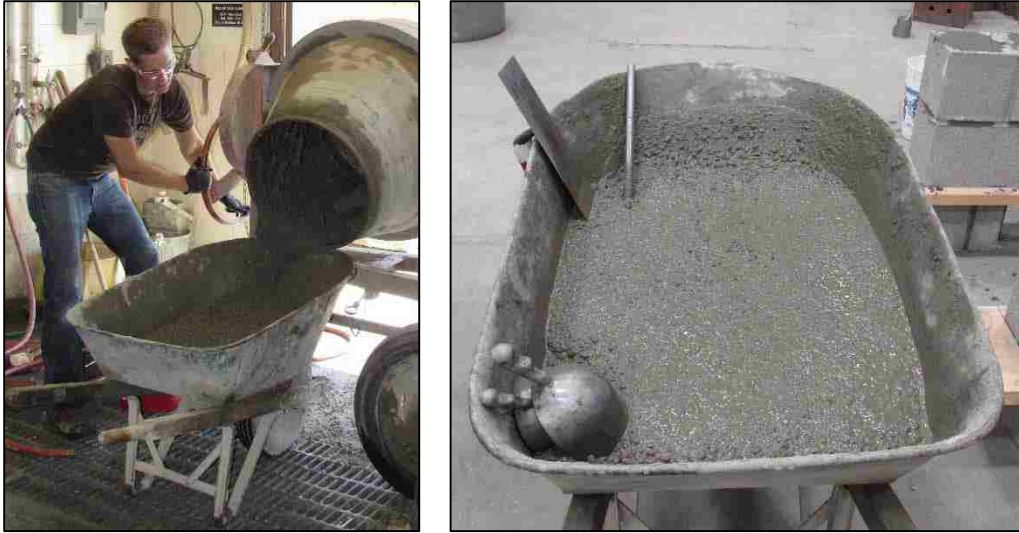
Figure 15. Grout Mixing and Composition
