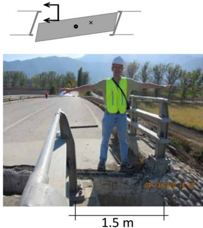
Figure 2-19. Bridge superstructure translation (Elnashi et al. 2010).
